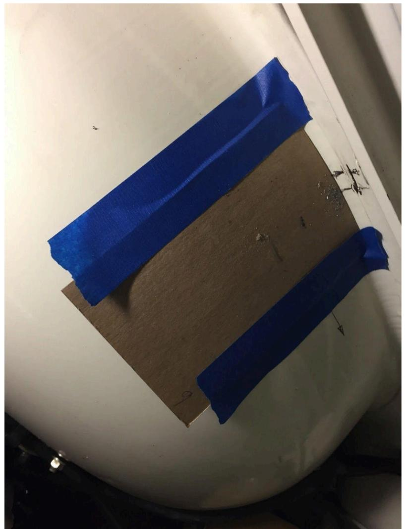
5. Drill carefully first with a small bit--1/16 or 3/32 inch--for accuracy. Then follow with 1/4 inch bit.
