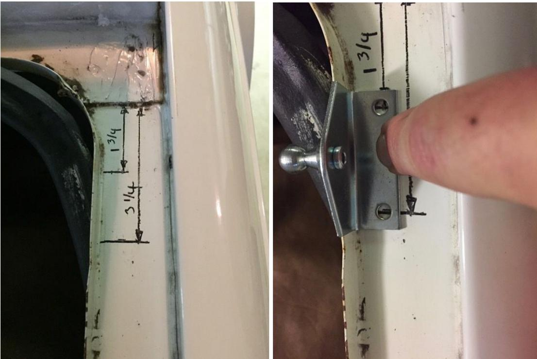
7. Find the proper drill points by using the lower bracket as a template and pressing your pencil INWARD as shown, while dragging the bracket along the standing metal edge.
